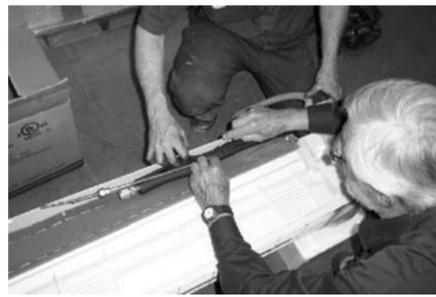
Slice the insulation before bending.
