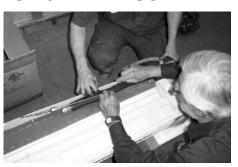
Slice the insulation before bending
